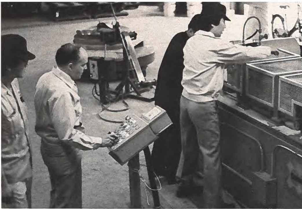
At control panel, Cominco engineer Ted Seymour, supervises installation of the Cominco Rotary Expander at a battery company in Japan.
