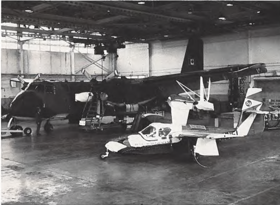
Lake LA-4 and de Havilland Buffalo with air cushion landing gear.
