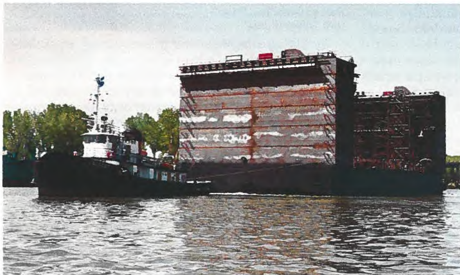
Seven sections of the PANAMAX drydock were assembled at the Tracey, Sorel, yards and floated down to the junction of the Richelieu and St. Lawrence rivers on its way to Halifax.
