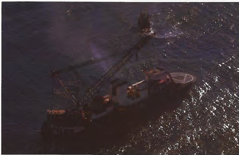
Pipe-laying vessels laying underwater pipeline to bring gas from Australia's North West Shelf gas fields to shore.
