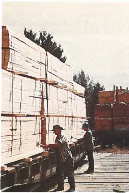
With increased house construction, lumber industry should improve.
