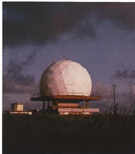
Airport Surveillance Radar at Grantley Adams International Airport, Barbados.
