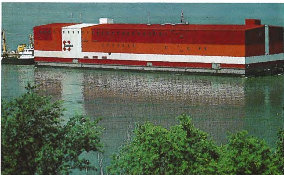
In another one of many joint ventures, DB-S and Comstock built the Cominco lead-zinc processing plant for Betchel. It was erected on a barge at Trois-Rivières and transported 2 500 nautical miles to Little Cornwallis in the Arctic.
