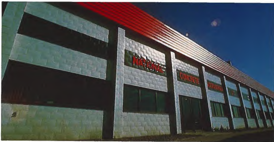
The National Concrete Accessories Warehouse in Calgary, Alberta, is an example of Mod-Lok exterior wall.
