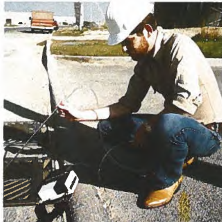
Armstrong's new portable amc 3000 detector used on a manhole.
