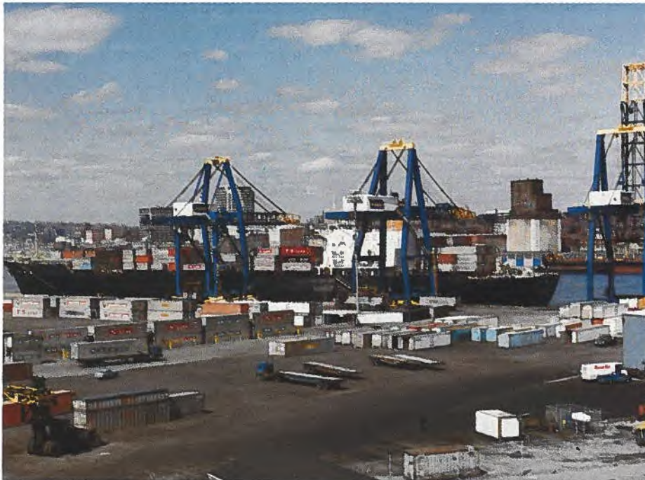
Vast and well-maintained loading areas are essential for container handling.
