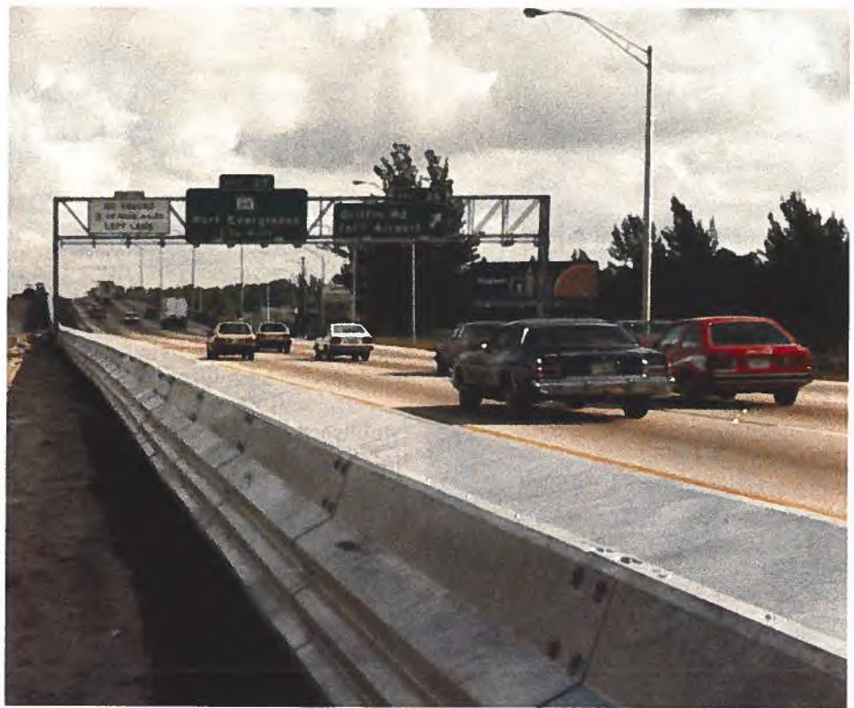
IBC Barrier in close-up.
