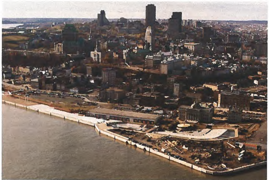
The "Old Port" under construction, summer 1983.
