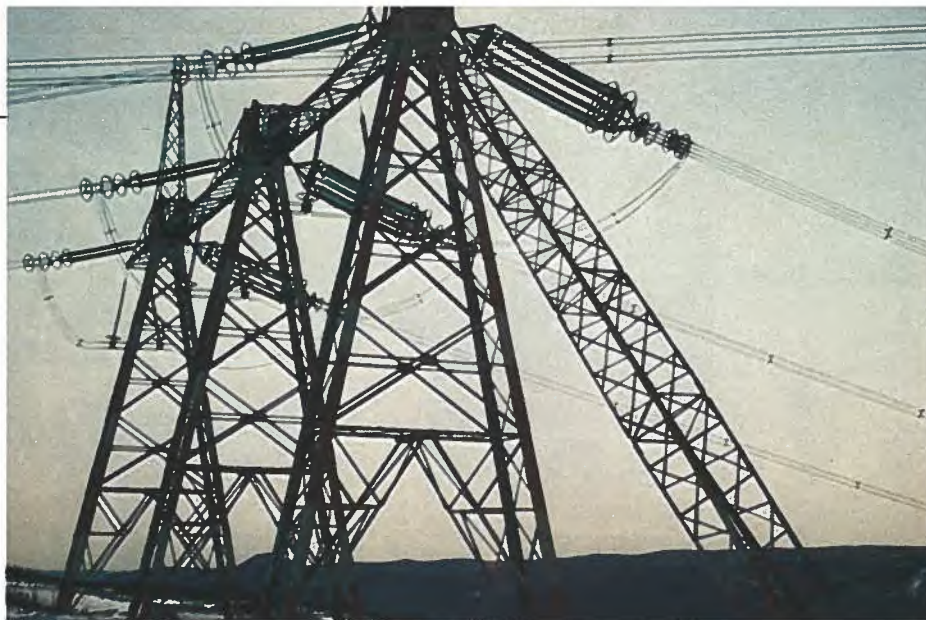
Power transmission towers, Churchill Falls, Labrador.
