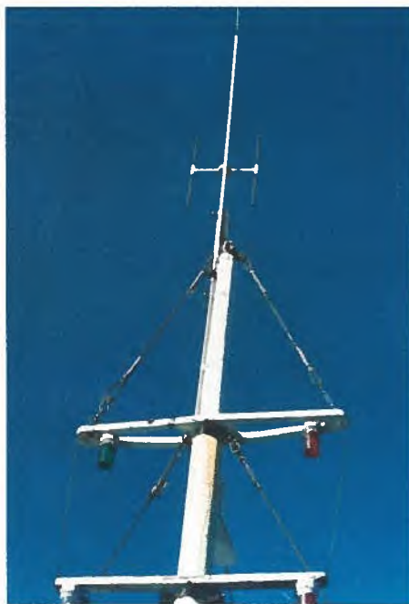
Ship's antenna — "H" near the top.
