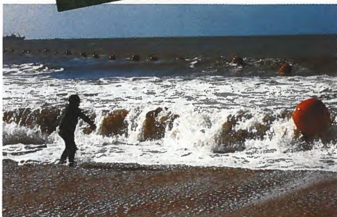
ANZCAN cable being floated ashore at Keawaula, Hawaii.
