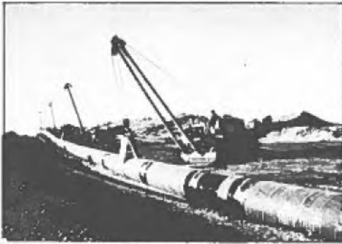
Construction of 42" pipe west of Sundre, Alberta
