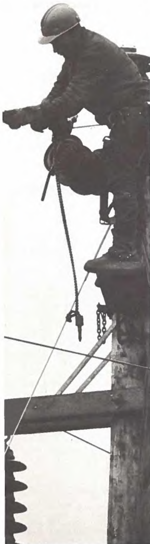
Hydro lineman at work, Churchill Falls, Labrador.
