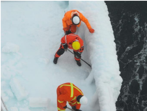
Figure 44 - Crew removing ice from bulwarks
