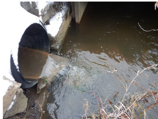
Picture 2: Untreated sewage flowed 325m along the length of the ditch into Lowden Brook. Enforcement officers collected samples and verified that it was deleterious to fish
