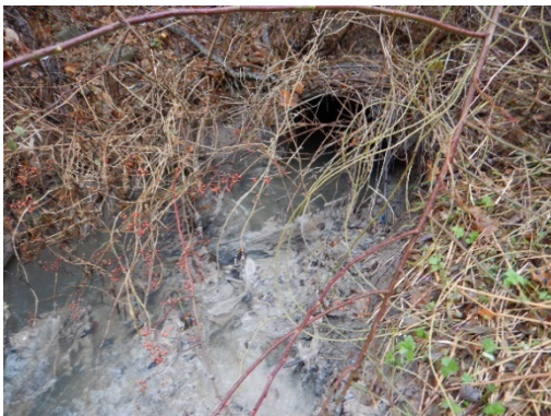
Picture 1: Untreated sewage overflowed into ditch due to blocked pipe
