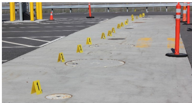
Picture 1: Overview of different manholes at the spill site
