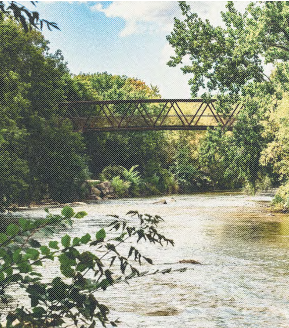
A wooden bridge crossing a river in Mississauga, Ontario, Canada, with trees and greenery along the banks.
