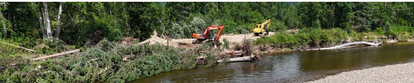
Side channel restoration. Raft River, BC. Courtesy of DFO staff.
