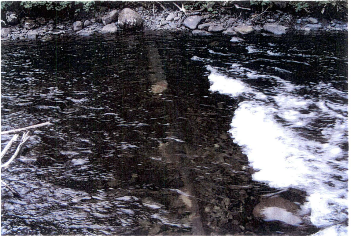
Photo 3. Sill rail/track installed in river at extreme low flow after weir removal.
