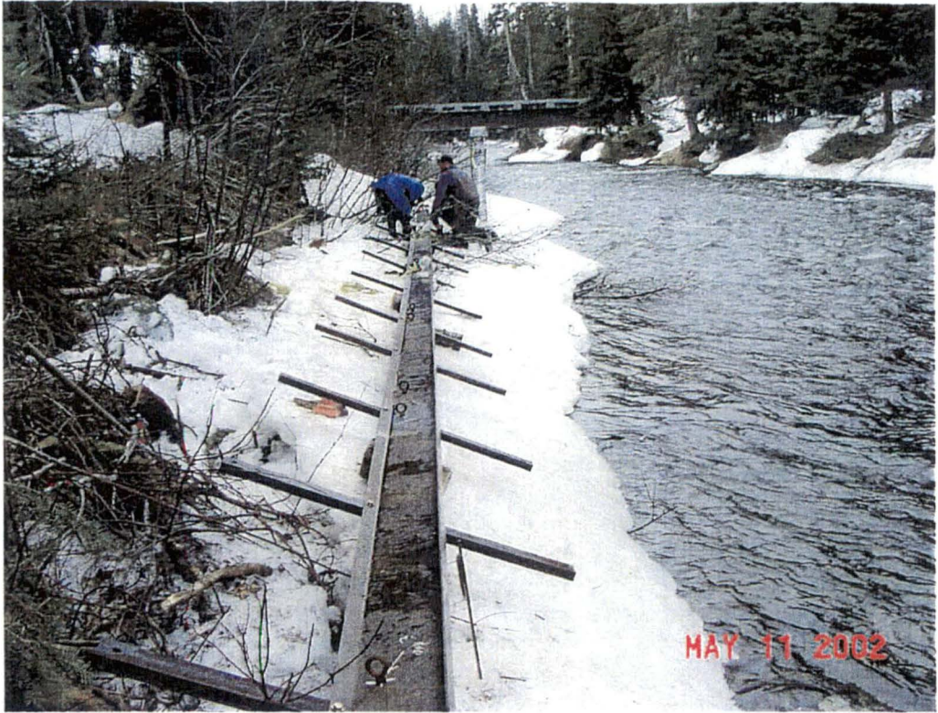
Photo 1. Complete sill rail/track before installation.
