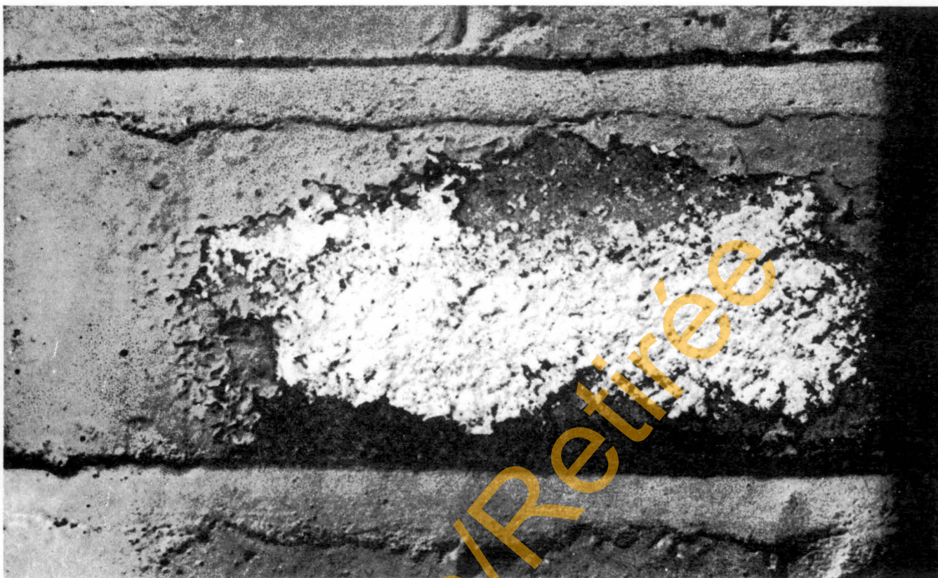
Efflorescence
