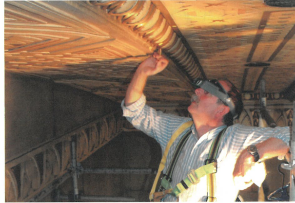
▲ CCI conducted an architectural paint study and cleaning tests on the vault of the former Bank of Montreal Building, Ottawa. 2
