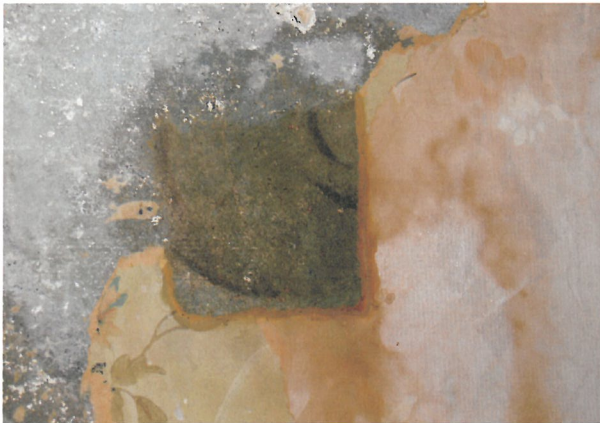
◀ Wallpaper removal tests were conducted on the south wall of the Painted Room at Sinclair Inn Museum, Annapolis Royal, Nova Scotia.
