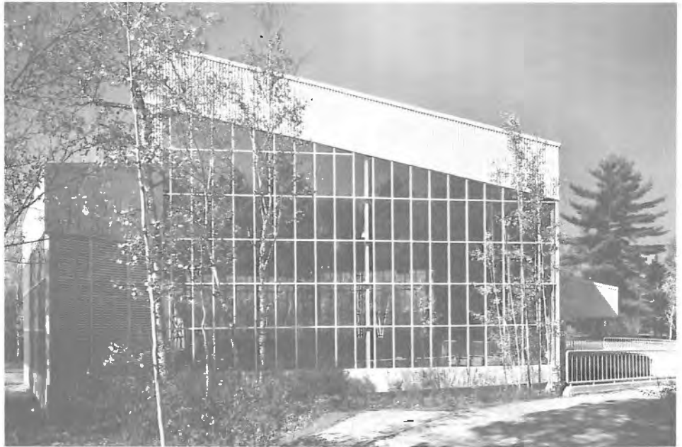
The southeast wall is entirely glazed to allow a maximum of sunshine on the marble surface and to make the outcrop partly visible as visitors approach it.
