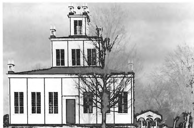
Figure 1. The Sharon Temple from the west. The square windowed towers that rise above the roof line are lanterns, which contain sconces for candles. A gold ball is hanging on four chains between the four upper lanterns. In the background is David Willson's study.
