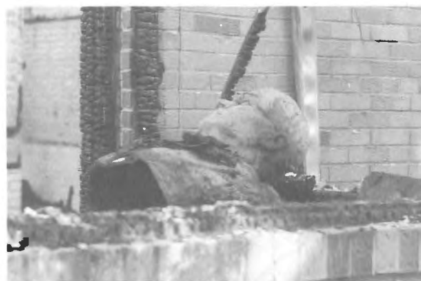
Figure 1. Taras H. Shevchenko Museum fire, Oakville, Ontario, September 1988.
