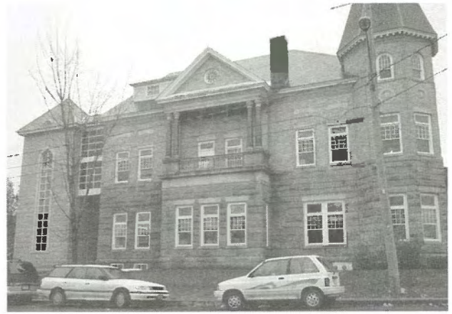
Exterior view of the Haskell Opera House (the left side is in Canada and the right side is in the United States).
