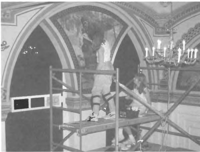
Helen McKay (left) and Debra Daly Hartin clean and consolidate a painting on canvas adhered directly to the wall in the Centre Block on Parliament Hill, Ottawa.
