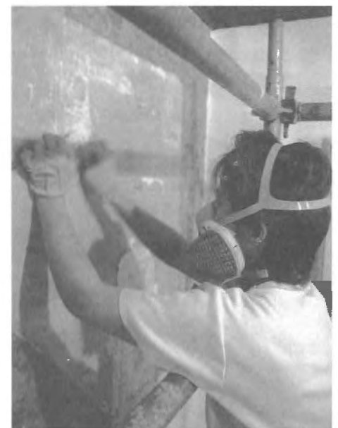
Holly Fiedler removing upper layers of overpaint after the application of solvent compresses.
