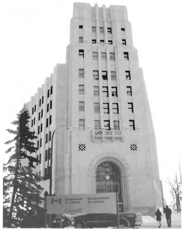
The Federal (Dominion Public) Building, Winnipeg, was built in 1937 in a modern Gothic style and is sited on an angular-shaped lot.
