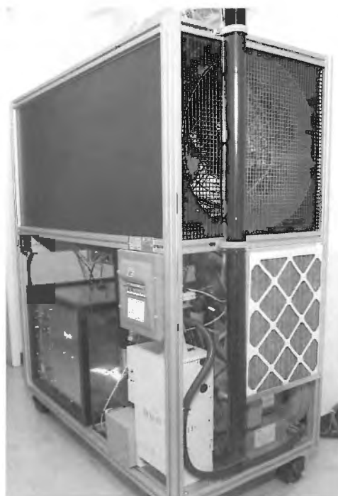
Figure 4. RH Control Module installation No. 2 at the Canada Science and Technology Museum. Serves the main exhibit area of the museum and is housed in what was formerly a small kitchen area. Provides controlled environments to artifacts in a display case at a fraction of the cost of proposed building-level systems due to a much lower airflow requirement (for cases). Eliminates the need to modify or upgrade the building envelope.
