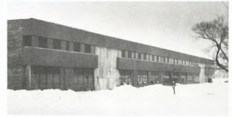
C.C.I. headquarters building during construction - exterior (Photo: W. Bokman)
