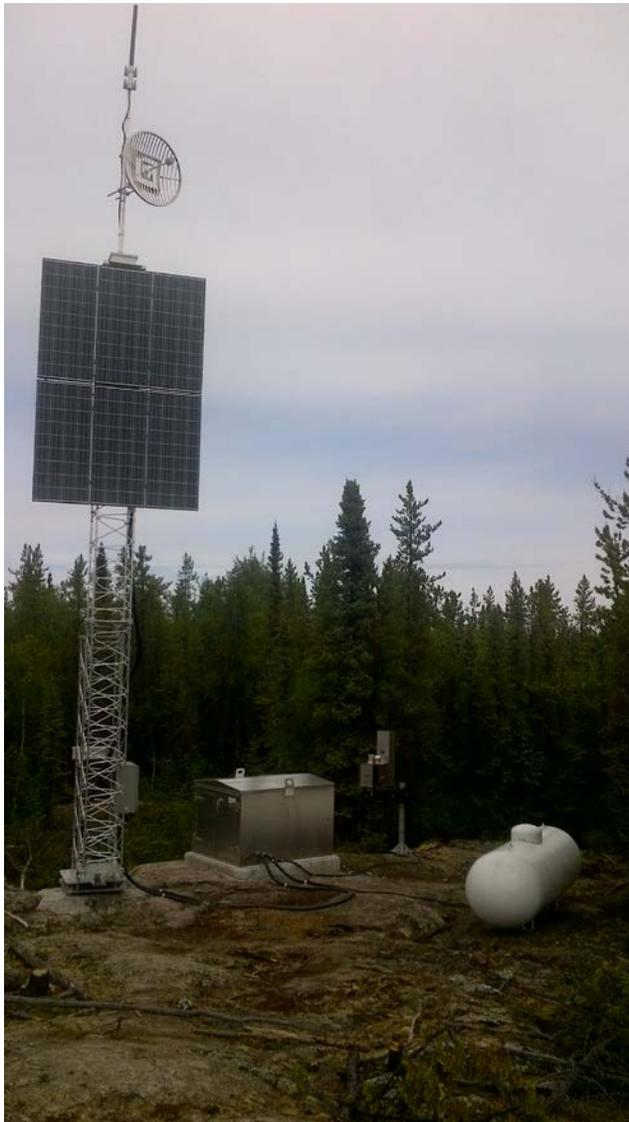
**Fig. 9:** Hybrid Solar-TEG remote power system for the Yellowknife seismic array stations. Six solar panels are mounted upon a 25' (7.62 m) articulated tower (left) and charge a bank of batteries (left of center) to power the station. A thermal electric generator (TEG, right of center) is used during later winter months when sunlight is unavailable, using propane (right) as its fuel source. The tower also provides a platform for the communications antenna.
