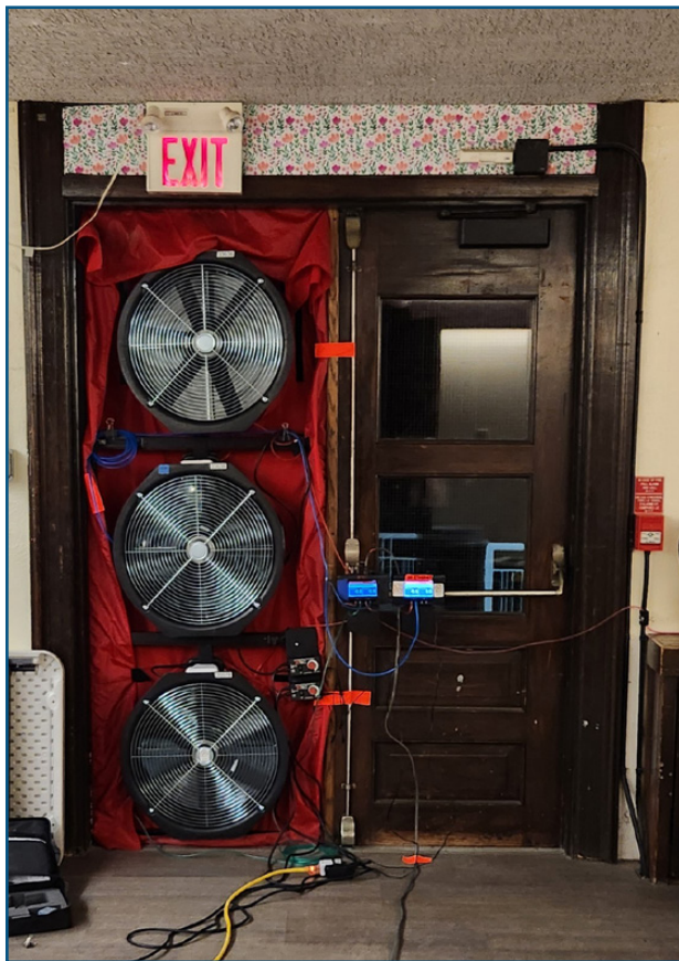
Figure 21: Power supply for blower door fans
