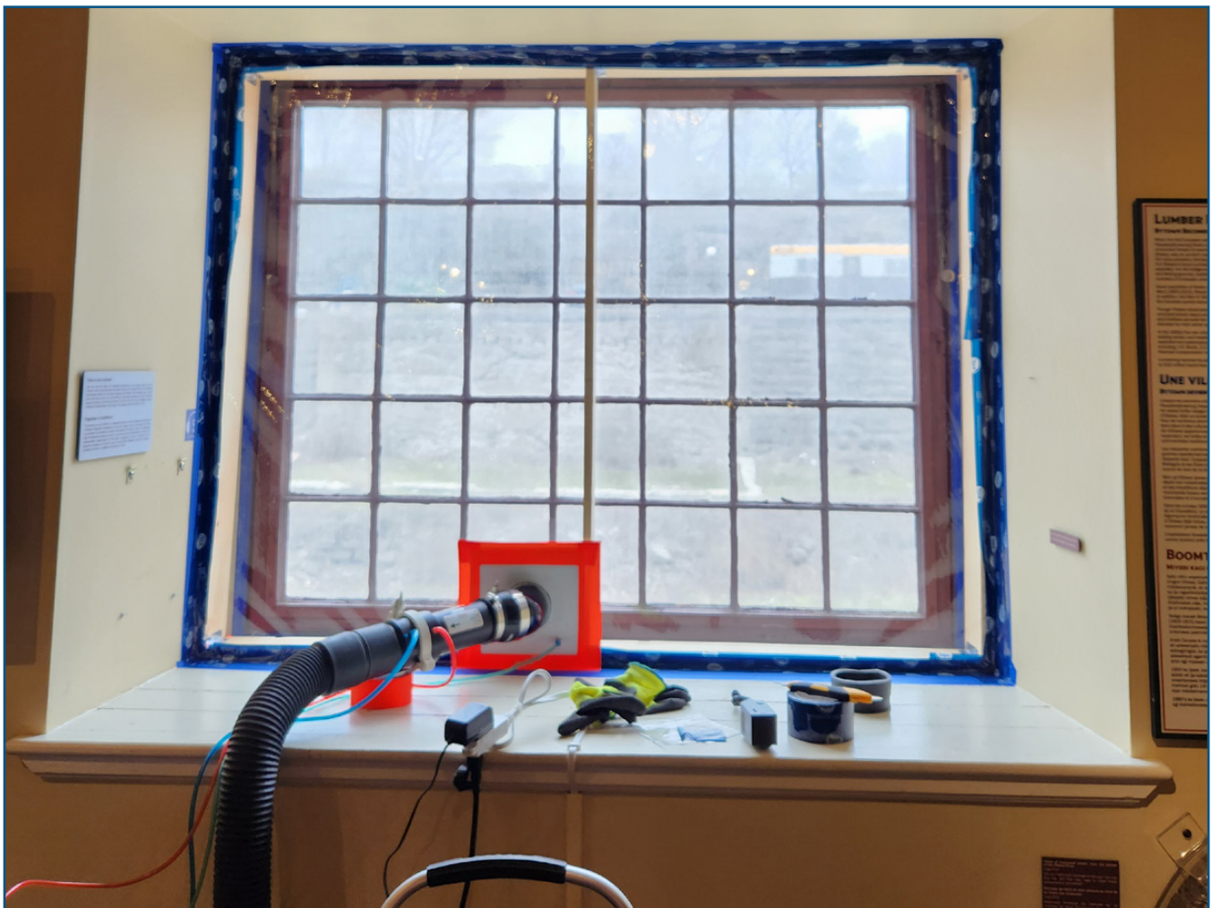
Figure 13: Localized component testing
