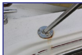
Rust at or on fittings
