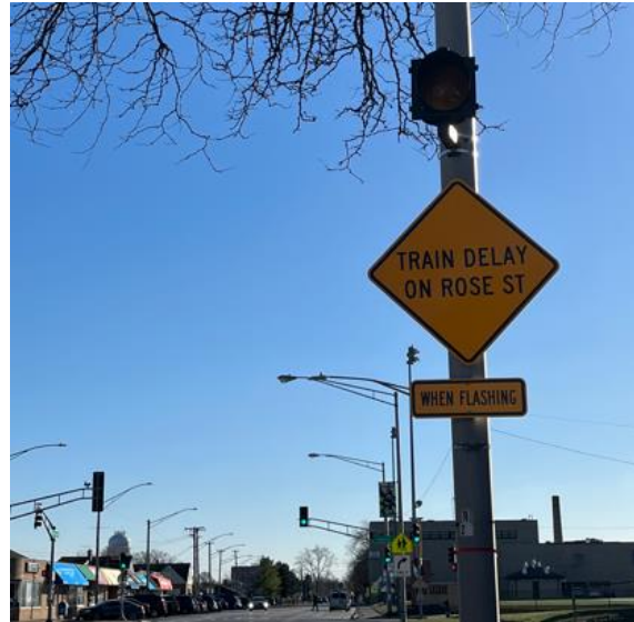
Figure 4: TRINFO Deployed Flashing Beacon
